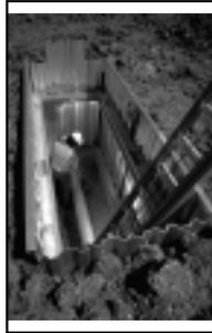
**End Panels:** Pre-engineered "end-panels" may be quickly attached to any Shoring Shield for 3 or 4-sided shielding.
