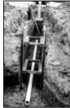
Unique end-loading capability allows for 3 and 4-sided protection.
