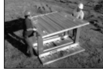
Attach hydraulic quick-connects to each Speed Strut. Lift top sidewall into position. Note: Machine assistance may be required on larger models.
