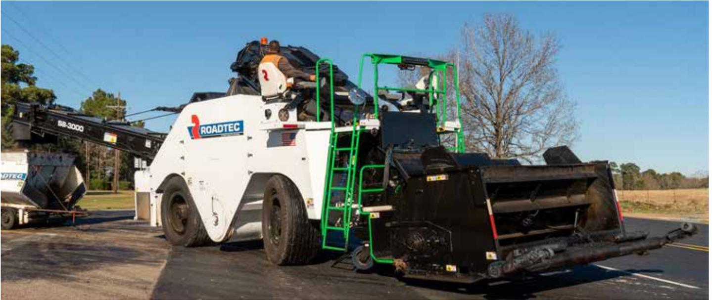
*In the photo above, an intersection is being paved, however, the dump truck is not able to maneuver into the intersection. Therefore, the mix is deposited from the dump truck into the hopper of the SB-3000 and shuttled to the intersection where the mix is deposited into the waiting paver.*
