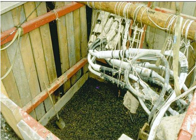
Manhole Braces, used in conjunction with appropriate sheeting, provide the active support necessary to secure safe excavations in less stable soils. Available in a wide variety of sizes and capacities, Manhole Braces are composed of modular sections for ease of assembly and transport. Manhole Braces feature 4-way hydraulic support with high-yield telescoping steel sections, and 4-way hose bridles for simultaneous
