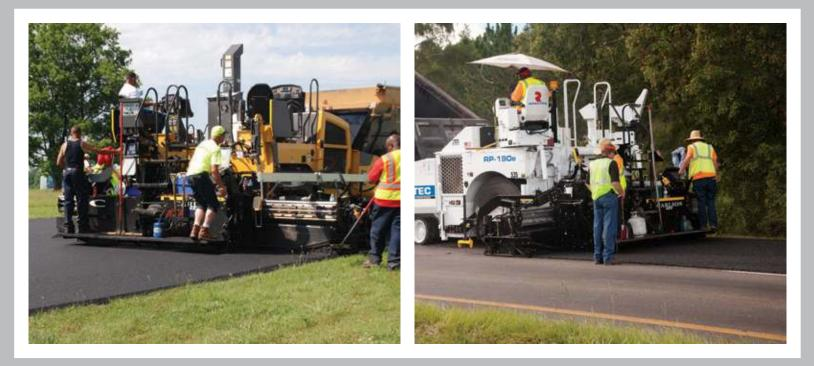
**Unmatched Performance** with its equal width single slide extensions, heavy duty extruded aluminum frame between the chrome rods for industry-leading strength, and class-exclusive ability to pave as a fixed width screed up to 30' (9.1m).
